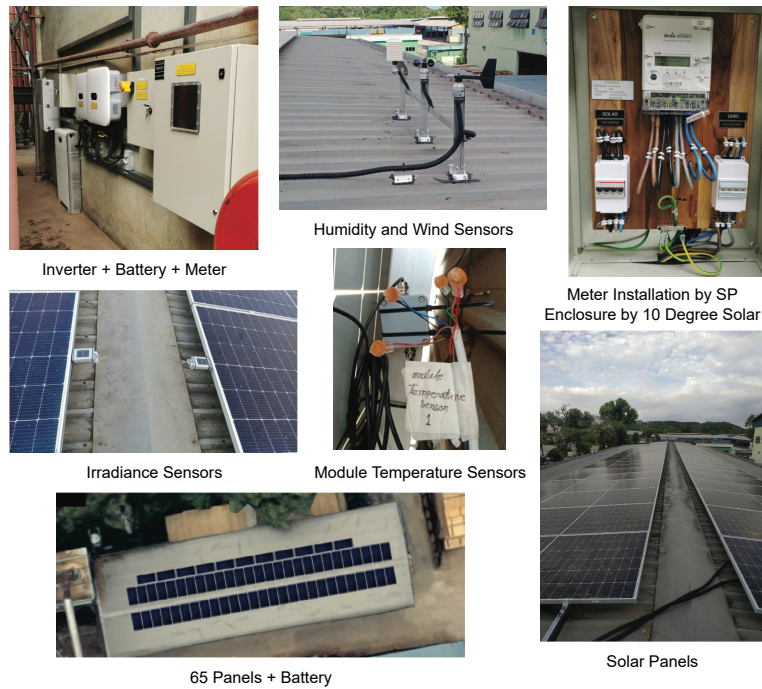
Figure 7: LHT Holdings Solar PV system.
